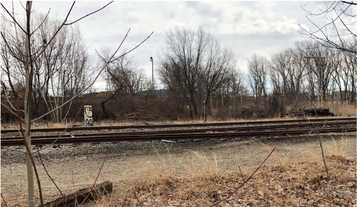
Photo A2. 4/4/23. The approximate crossing location of the bridge that would be constructed over the active CSX Railroad, view southeast.
