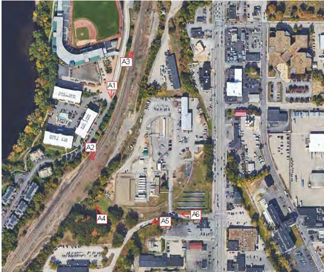
Google Earth photo of Element A area showing photo locations for S. Commercial Street Extension near Fisher Cats Stadium at upper left, across active rail corridor, and connecting to Gas Street. Liberty Utilities is in the center, and Elm Street runs north to south just east of Liberty Utilities.
