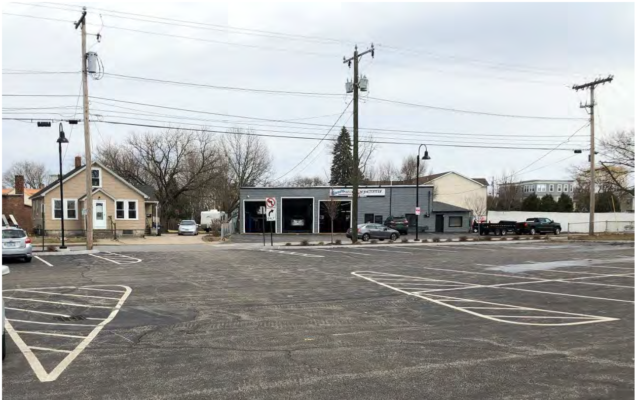
Photo C7. 4/4/23. The location where Gas Street Extension would reach South Elm Street, view east.
