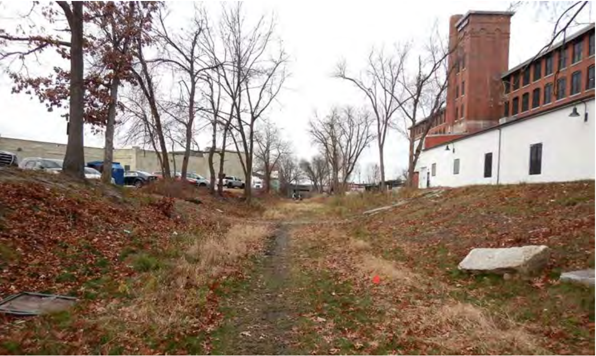
Photo C4. 11/29/22. View of the abandoned railroad bed behind the Cohas Shoe Factory building, where the bridge would be constructed, looking north-northwest.
