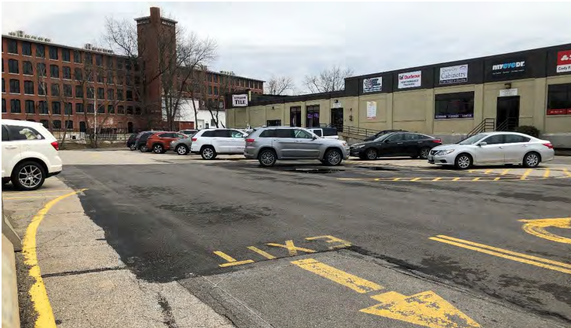
Photo C1. 4/4/23. View southeast where new Gas Street Extension would pass through an existing parking area along the east side of Elm Street towards the Factory on Elm.
