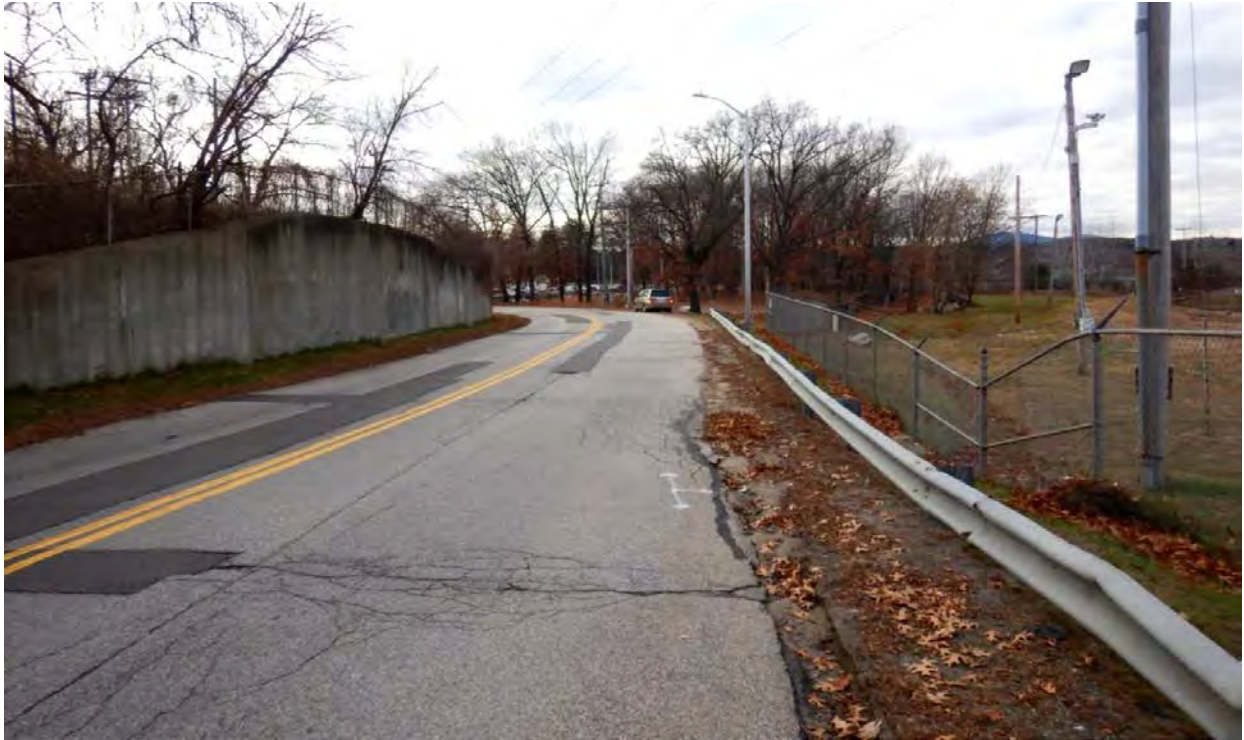
Photo A5. 11/29/22. View of Gas Street where improvements will be made, facing west-southwest.
