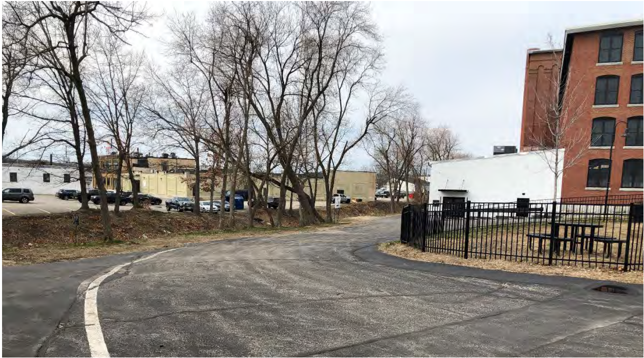
Photo C6. 4/4/23. Proposed Gas Street Extension location east of the abandoned rail corridor, view northwest
