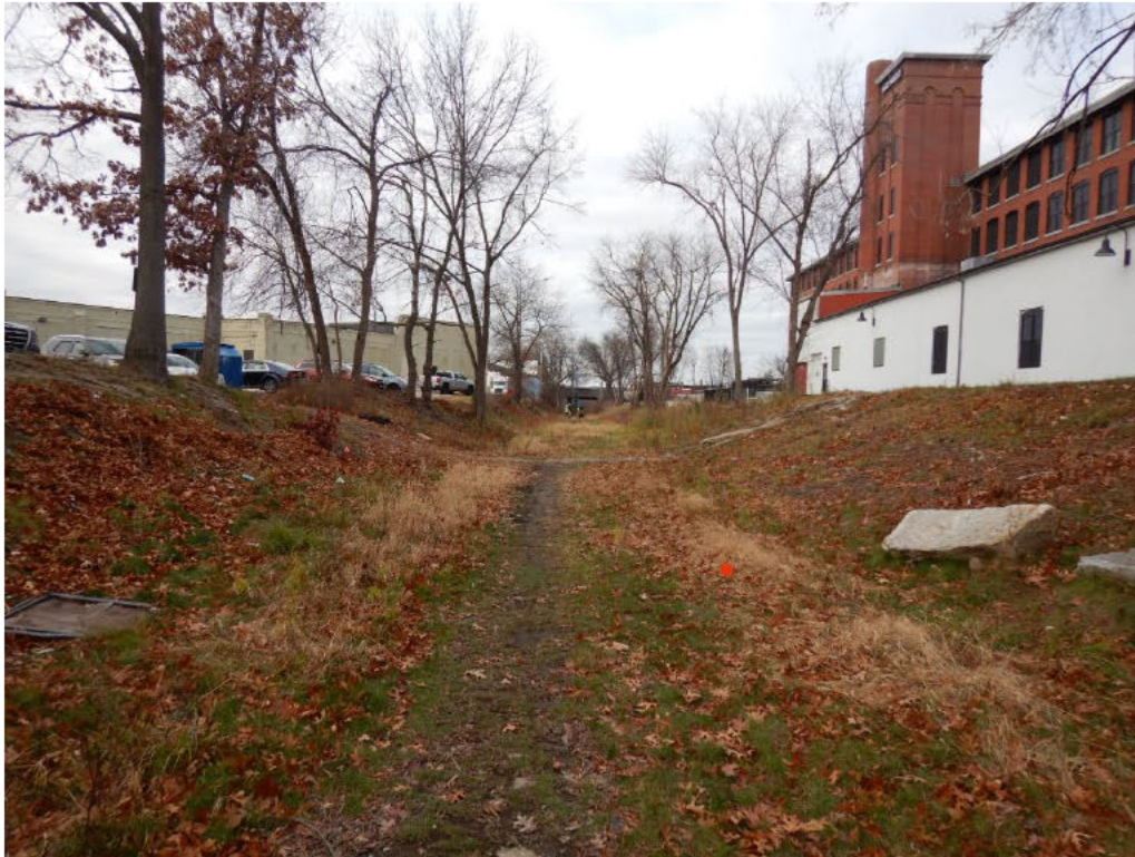
Photo 12. View of the abandoned railroad bed running behind the Cohas Shoe Factory building (right). Note the slope of the ground on either side, indicating that the ground was lowered to create a level surface for the railbed. View facing northwest.
