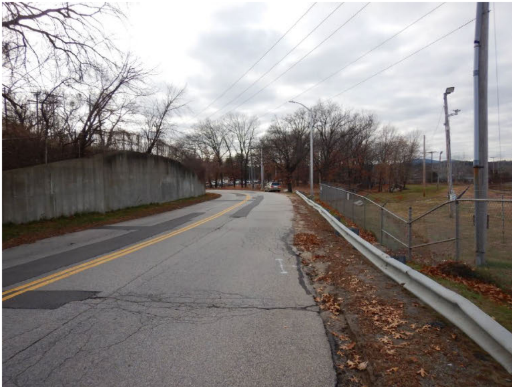
Photo 5. View of Gas Street. Note the large concrete retaining wall (left) which shows that a substantial area of the hillside was removed when Gas Street was built. View facing west-southwest.
