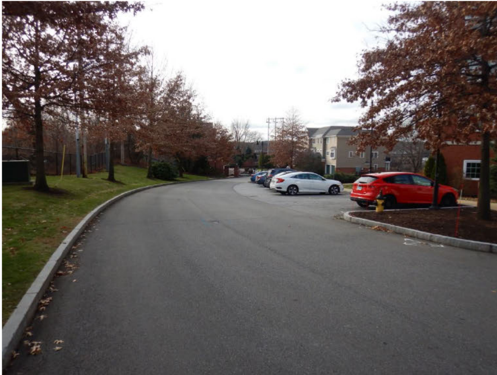
Photo 2. The curved portion of Riverwalk Way. Note the landscaping with deciduous trees, utility box, and electric poles (upper left). Also note the slope of the ground on the shoulder compared to the road's level path, indicating that the landscape was graded to create the road. View facing southwest.
