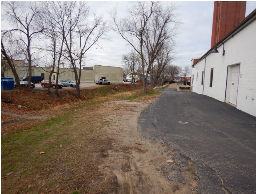
Photo 14. View of the railbed from the ground level of the Cohas Shoe Factory. Note the pronounced steep slopes down to the railbed. View facing northwest.
