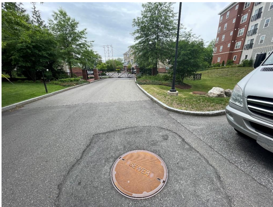
Area F: View of sewer service along South Commercial Street.
