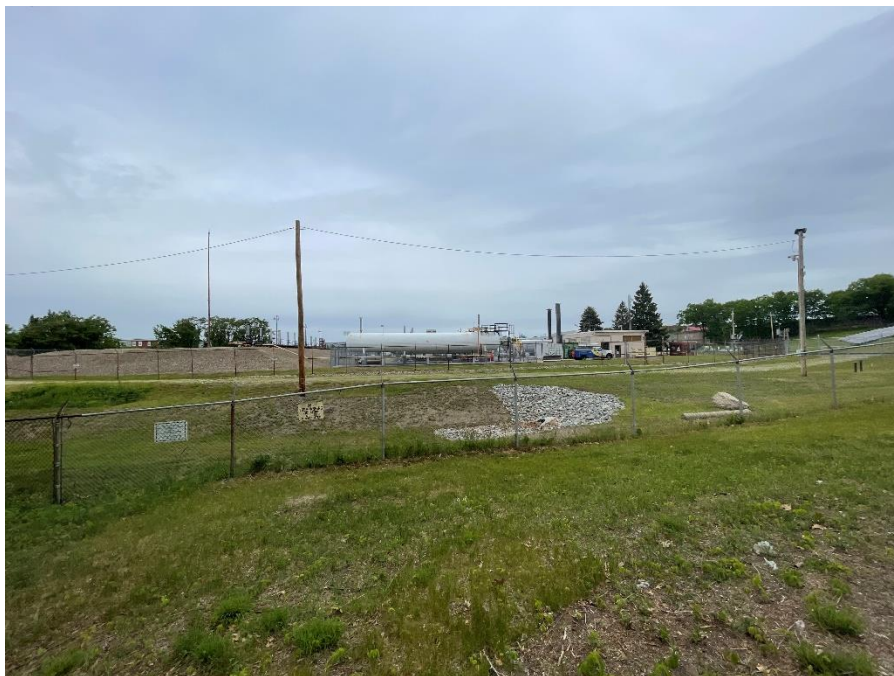
Area F: View of Liberty Utilities located north along Gas Street.
