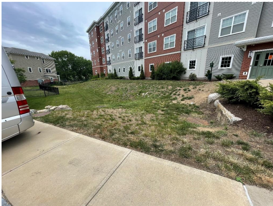
Area F: View of drainage network west of South Commercial Street.
