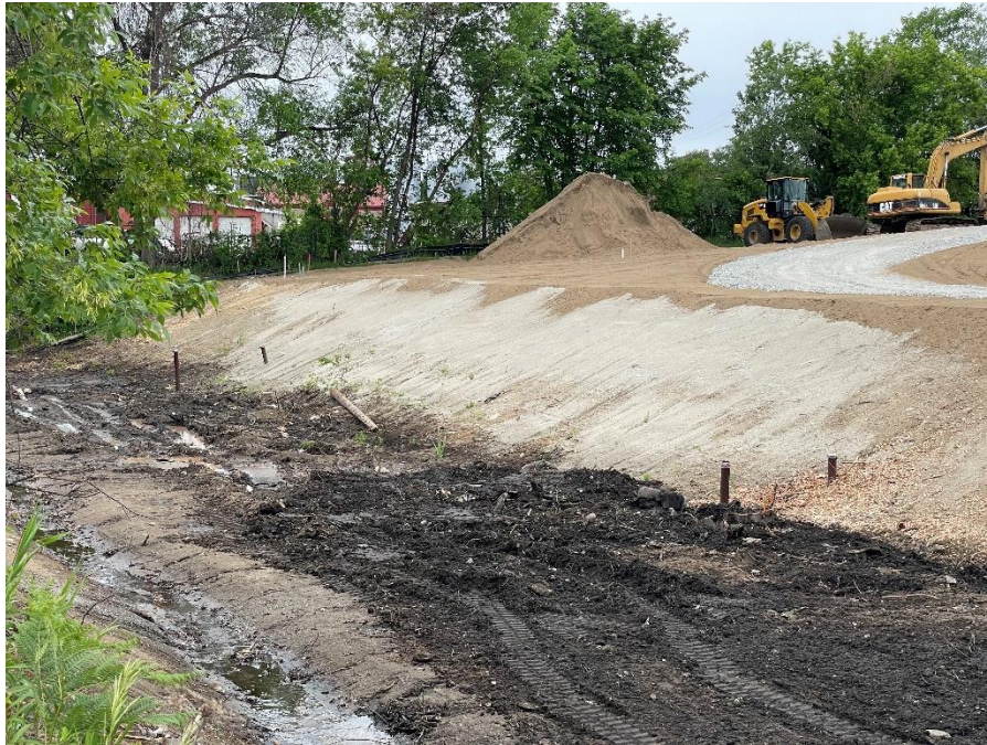
Area C: View of the railroad corridor with monitoring wells, from Elm Street after under passing the Elm Street Bridge, facing north.
