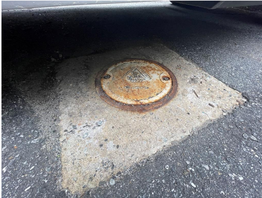
Area F: View of monitoring well observed in the parking lot of the Residences at Riverwalk.
